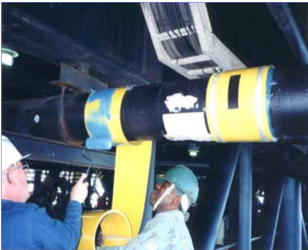
Figure 13. Offshore application of a 'Clockspring' repair to an externally corroded pipe (Courtesy of Clockspring Ltd).
