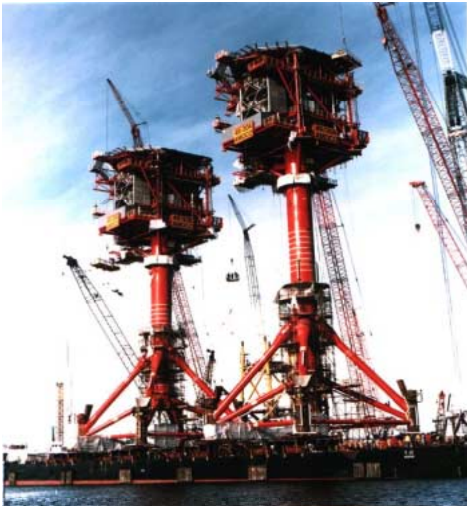
Figure 2 Davy and Bessemer monopod platforms, which contained 10% of composite materials in the topside structures (Courtesy of BP-Amoco).
