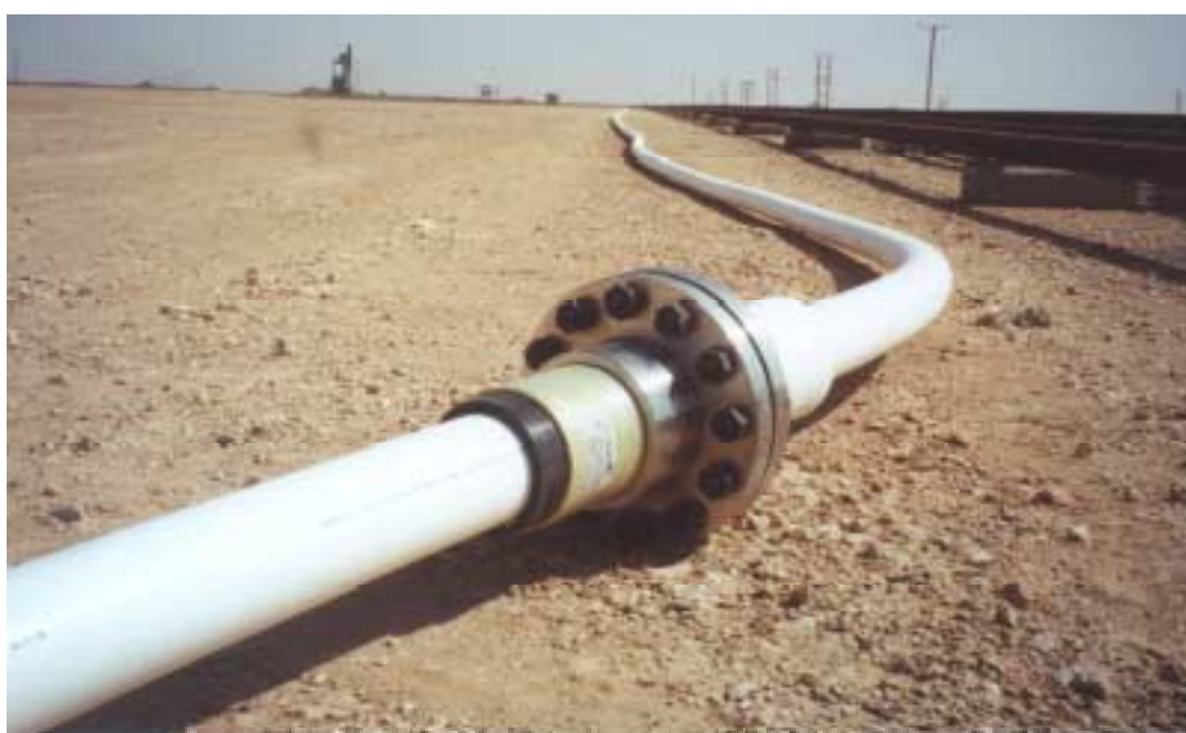
Figure 10. Field trial of RTP for oilfield fluids (Pipelife BV)..
