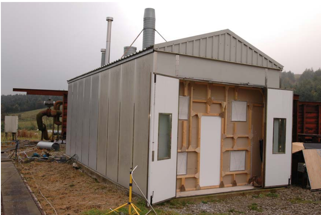
Figure 17. Spray room configuration 2 (Experiments 21 and 22) – showing back wall and filter panels
