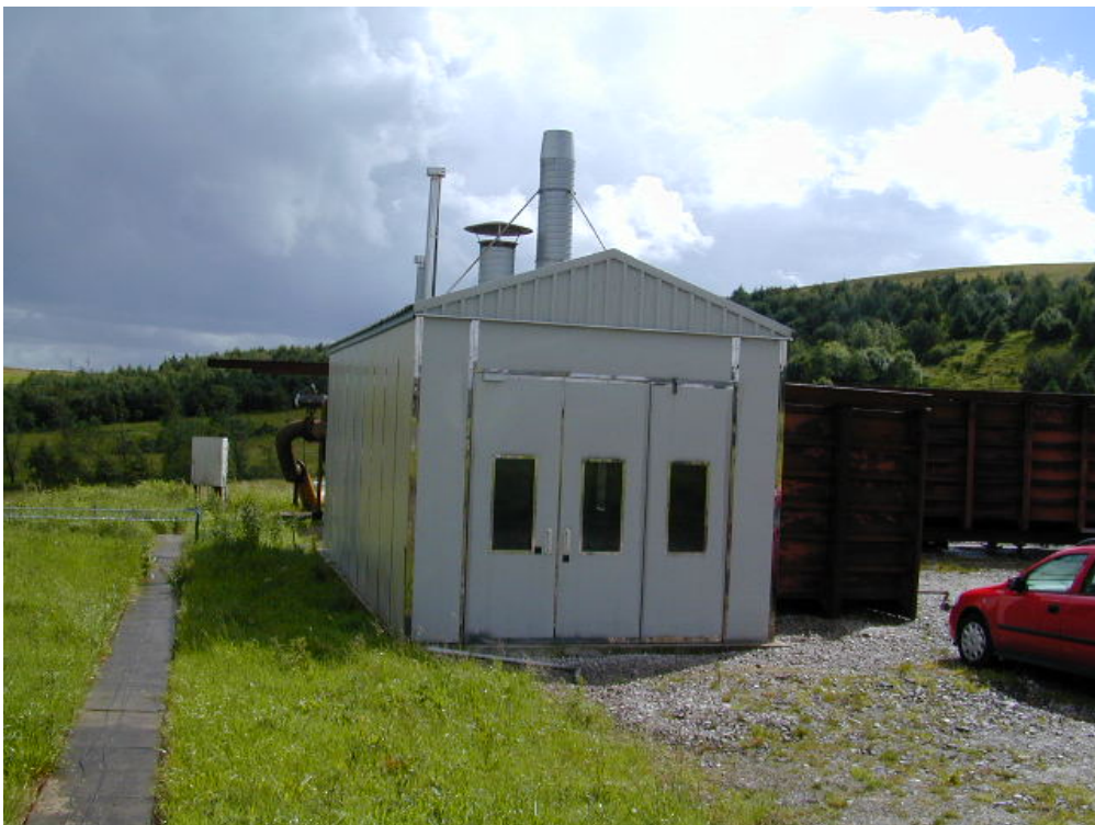
Figure 12. HSL Spray Booth
