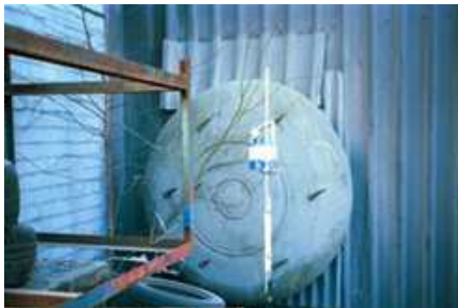
Figure 5. Cowl fitted to the outside of the axial fan
