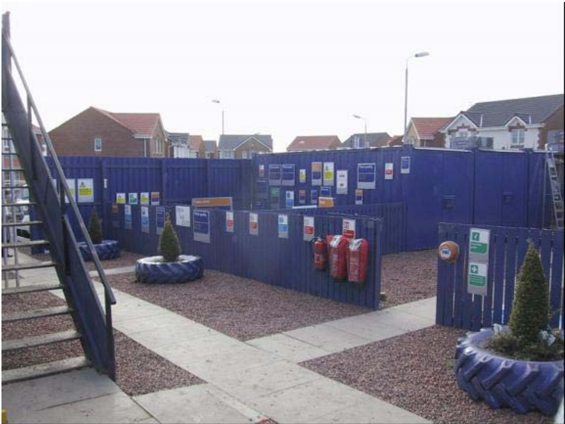
Figure 2 Health and Safety messages on a construction site
